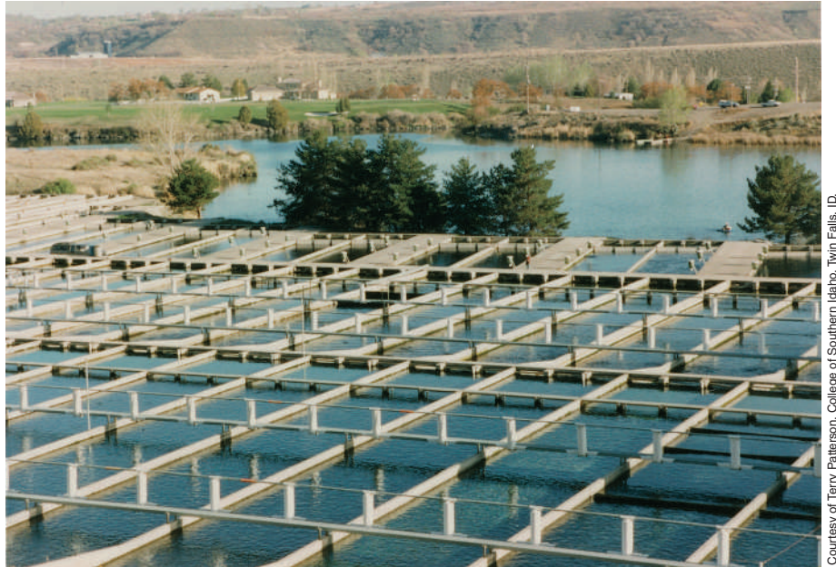
FIGURE 13-12 Raceways at the world's largest commercial trout production facility, Clear Springs in Buhl, Idaho.
