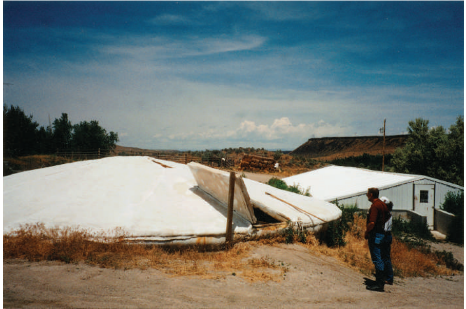
FIGURE 8-3 Alligator grow-out facility built into the ground to conserve heat.
