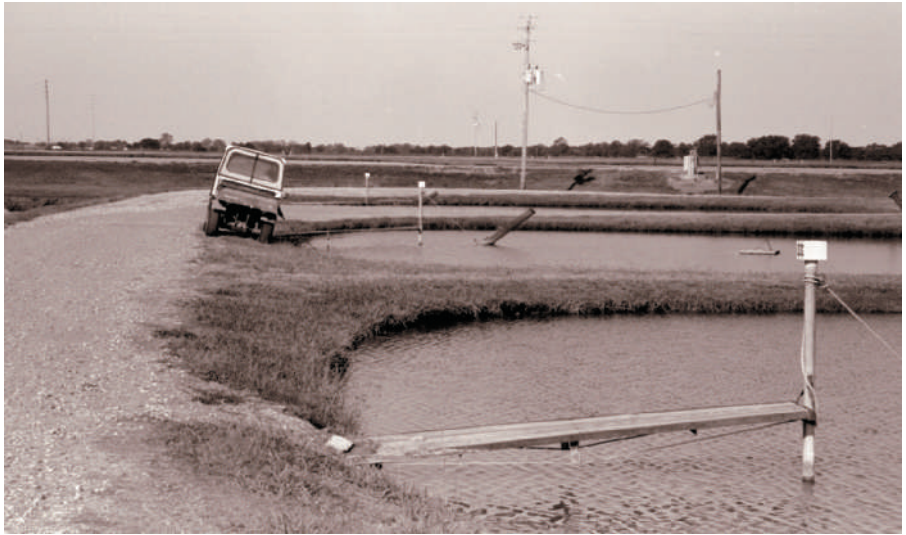
FIGURE 13-10 The modified Canfield outlet or inside swivel drain controls the water level by pivoting the drainpipe up or down on its swivel joint.
