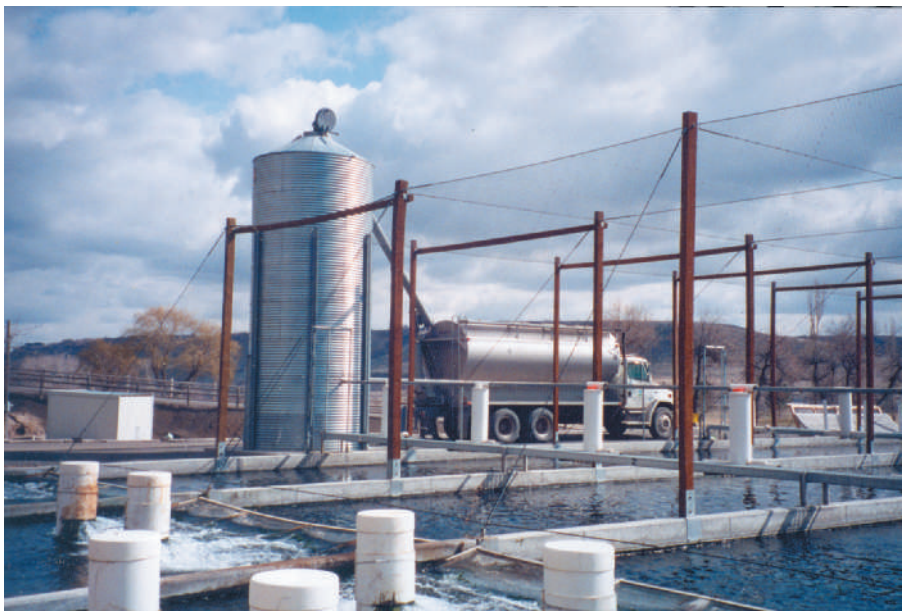
Figure 4-47 Wire netting used to keep birds out of trout raceways.
