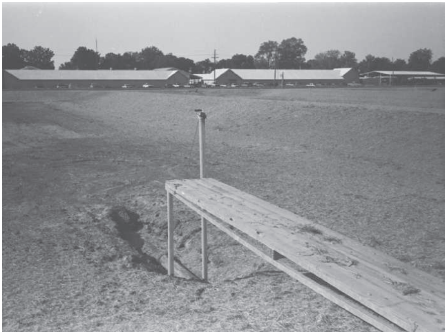
FIGURE 13-11 Swivel drain in a newly constructed pond. Pipe is lowered to drain the pond.
